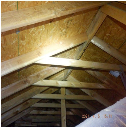
Attic Framing/Sheathing: Framing/Sheathing
