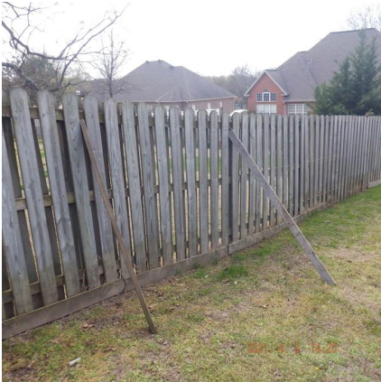
FENCES / GATES: Broken Fence Posts
