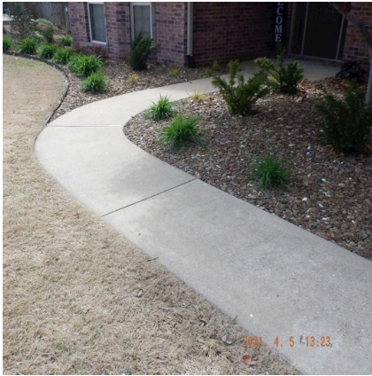
Walks / Steps: Walkway
