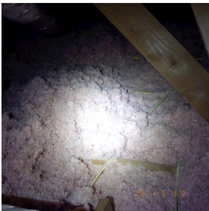
Attic Insulation: Loose Fill Insulation
