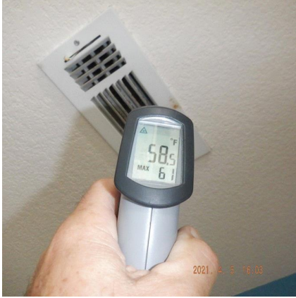
Cooling: Supply Air Temp
