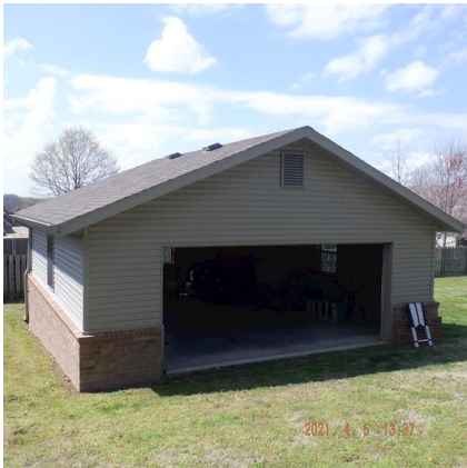
Exterior Structures - Shop: Shop
