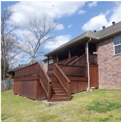
Decks / Balcony: Back Deck
