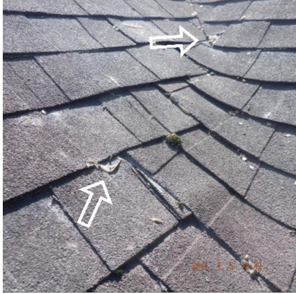
FLASHING/VALLEYS: Repairs In Valley
